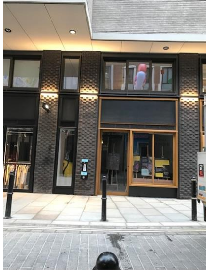
Ganton Street entrance and entrance slope
