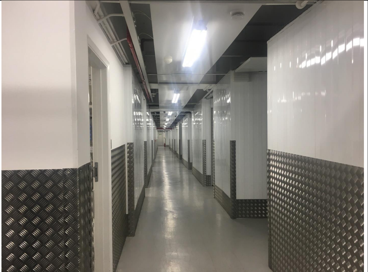
Existing self-service units at level 1 within the car park
